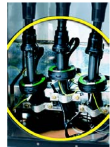
Opening core balance CT's
